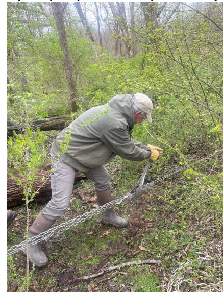
The pulling power comes from the guy working the come-along anchored to a nearby tree.
